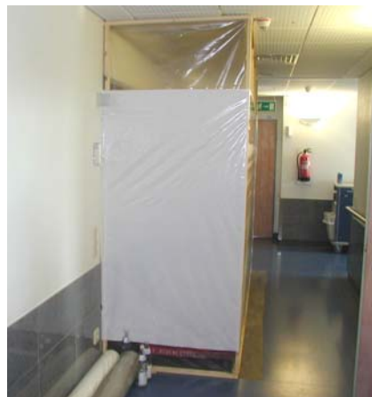
Plastic sheeting on wooden support around internal renovation, negative pressure
