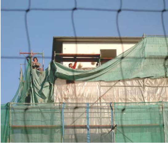
Erecting barrier around demolition work
