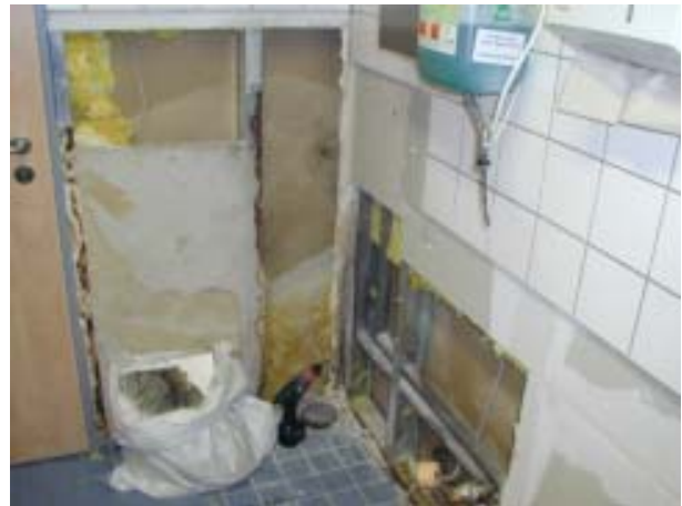
Water damage in disinfection room
