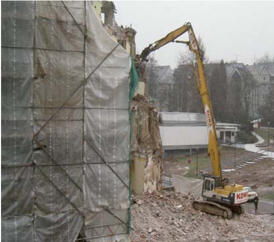
Erecting barrier around demolition work
