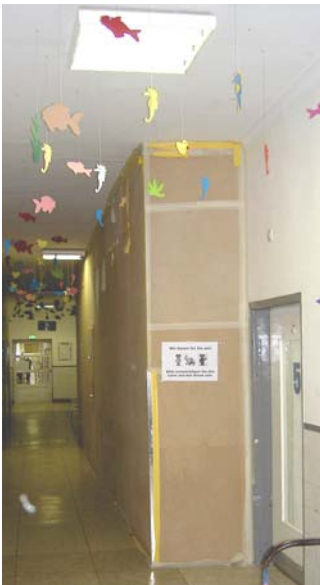
Solid barrier around internal renovation, seen from the clean side
